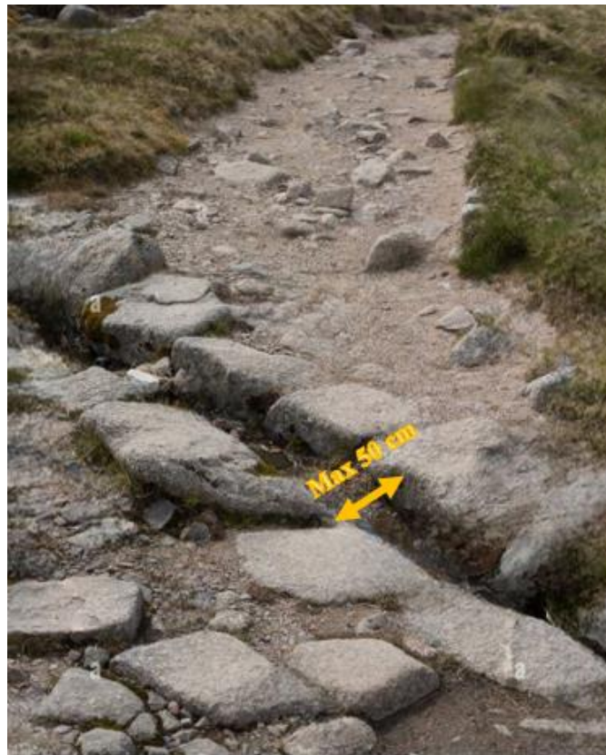
Figure C-17: Open cross drain
