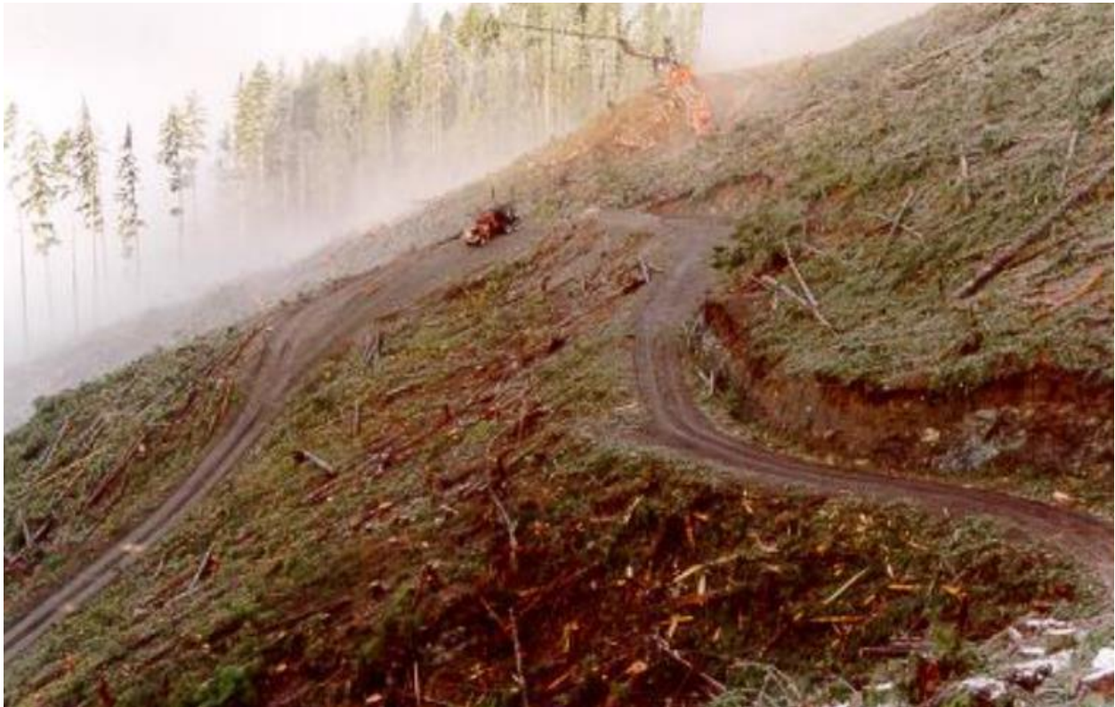
Figure D-12:- constructed switchback
