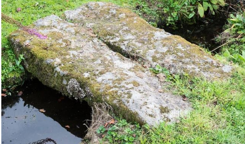
Figure C-20:- stone slab culvert
