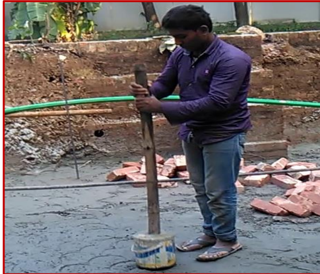
Figure C-5: Hand compaction
